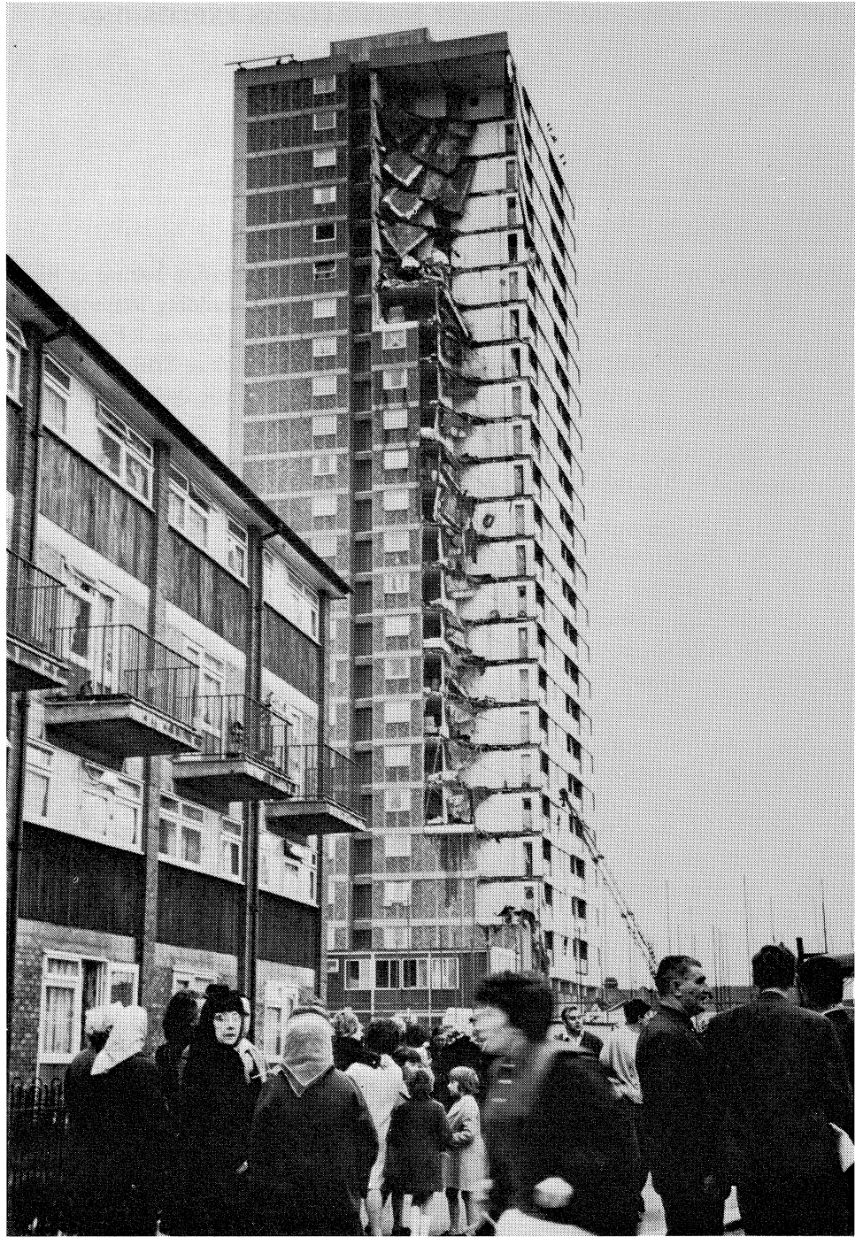
Fig. 1. Collapse of Ronan Point, a block of flat, as a results of an explosion of town gas in the corner flat on the 18th floor.
