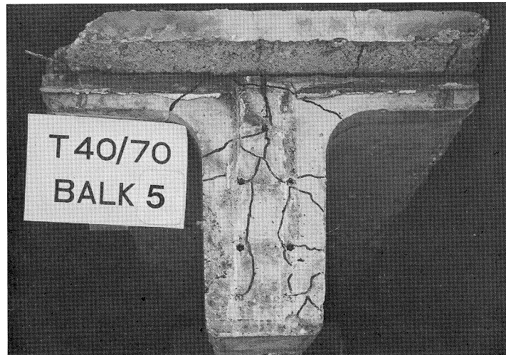
Fig. 5. Slip of 7-wire 12.5 mm strand in a T-beam exposed to fire along its entire length.
