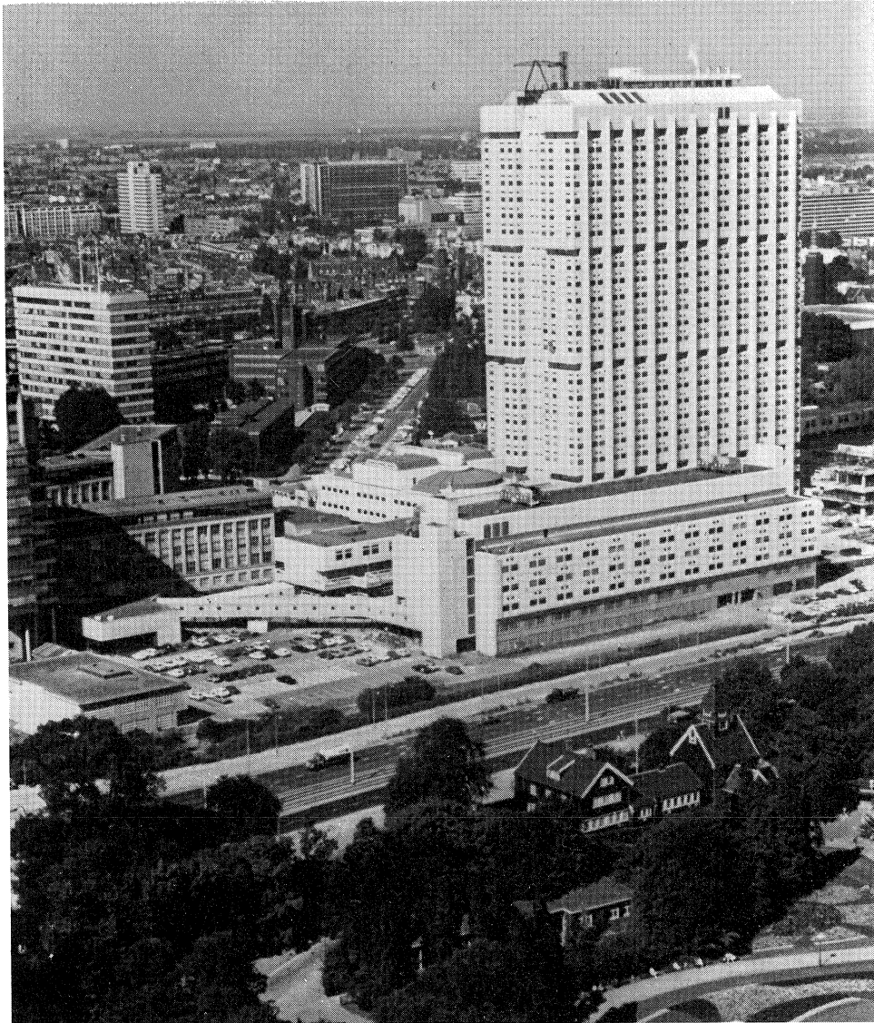
Fig. 51. Building of Erasmus University, medical faculty, Rotterdam.
