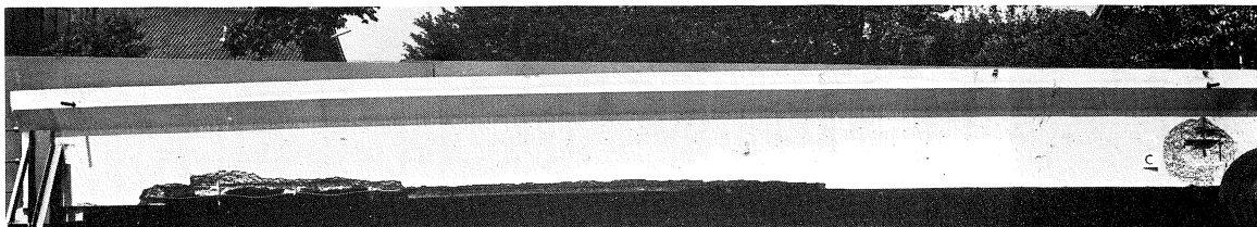
Fig. 2. Prestressed lightweight concrete beam after a fire test.
