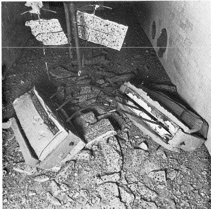
Fig. 42. Slab in series d after the fire test.
