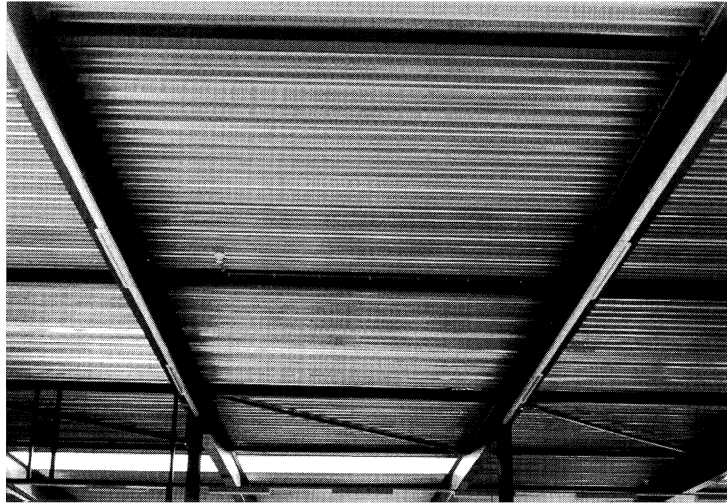
Fig. 1. Sheeting used for roof construction.
