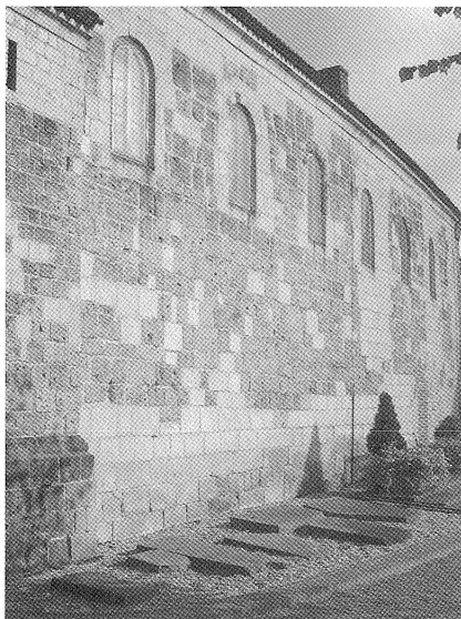
Fig. 3. Mixture of recycled Römer tuff and Weiberner tuff in the Old Church, Oosterbeek, rebuilt after serving as a British bridgehead in the late 2 nd World War.
