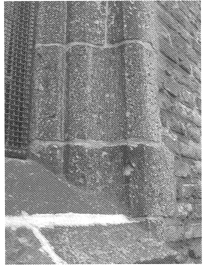
Fig. 14. Aveoli on Ettringer tuff, Old Church, Delft.
