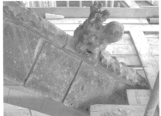
Fig. 2. Römer and Weiberner tuff on one of the rampant arches of St. John's cathedral, s Hertogenbosch, probably dating back to the 14 th – 15 th century.
