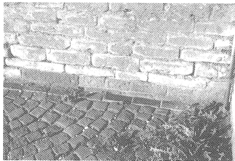
Fig. 19. Römer tuff with hard, glassy surface at street level below Gobertange sandy limestone of the St. Lambertus tower, Vught.
