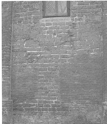
Fig. 1. Surviving 11 th century Römer tuff on the north façade of John's church, Utrecht.
