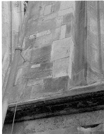
Fig. 1. Part of the façade of St. John's cathedral, 's Hertogenbosch, built in Bentheim sandstone. Note the variable intensity of black weathering. Samples Z1 and Z2 (Table 2) have been collected from this façade.
