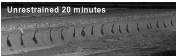
Figure 7. Thermal cracks in the web of a 200 mm deep slab after 20 minutes of fire exposure
