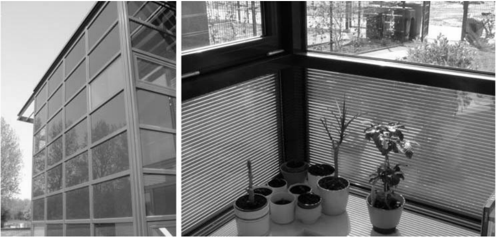
Figure 9: Example of solar energy systems in single skin; similar to glass facades
