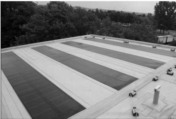
Figure 10: Application of flexible product in the outside building skin
