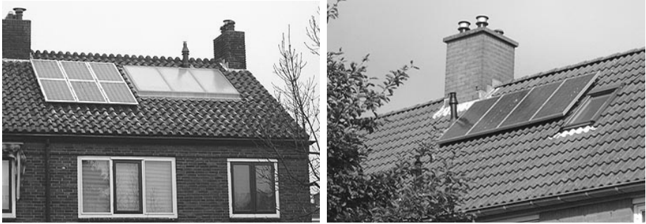
Figure 6: Examples of systems parallel to pitched roofs
