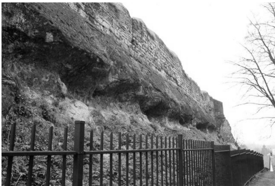
Figure 2. Ruin of Valkenburg castle (12th-17th century), with the remains of the surrounding wall in Maastricht limestone on top of that limestone itself. Decay of both the wall and the rock is clearly visible (2001)
