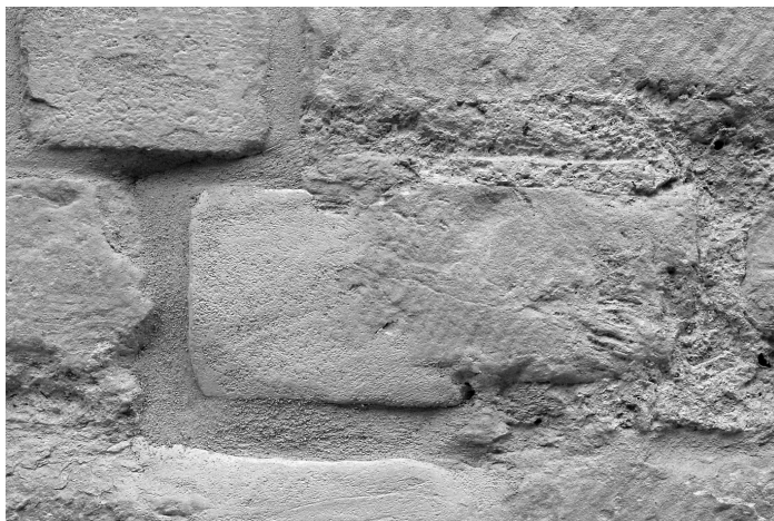
Figure 15: Compatible use of Monulit mortar. (photo: author)
