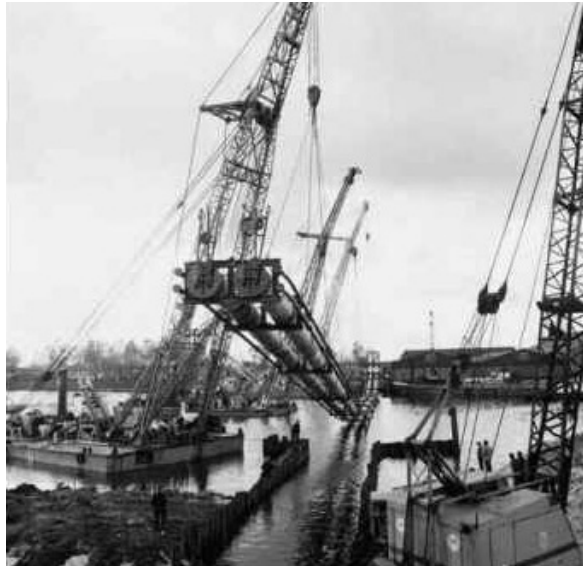
Figure 1: Pipeline crossing a canal (photo: ir. A.M. Gresnigt)
