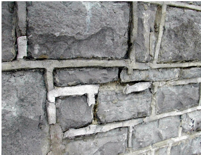
Figure 5. Push out of a dense repointing mortar caused by frost damage to the bedding mortar. Combination of problems: strong dense mortar (restricts drying, shrinkage cracks allow ingress of moisture); depth of the repointing insufficient (wrong on-site practice). Free-standing garden wall, Ottawa, Canada. (P. Maurenbrecher)
