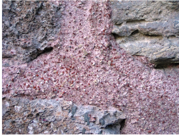
Figure 6. Mortar containing crushed brick particles as pozzolana (Istanbul)
