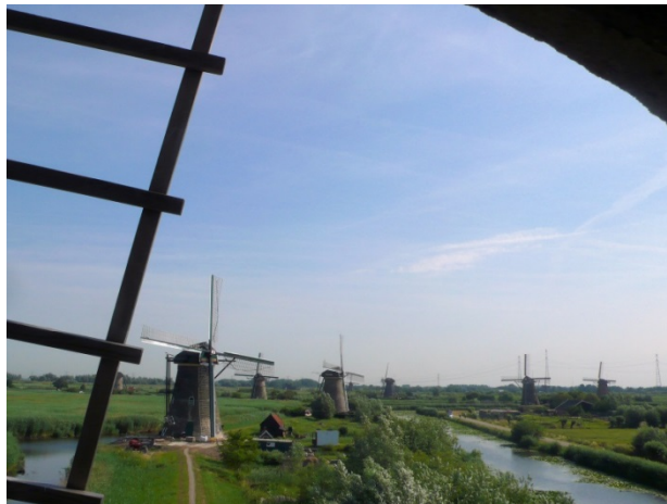
Figure 12. Water mills built in 1738 at Kinderdijk, the Netherlands. They are almost identical in design, but built by different contractors. Striking are the differences in quality of these mills. From the beginning several of them are suffering from serious rain penetration problems.
