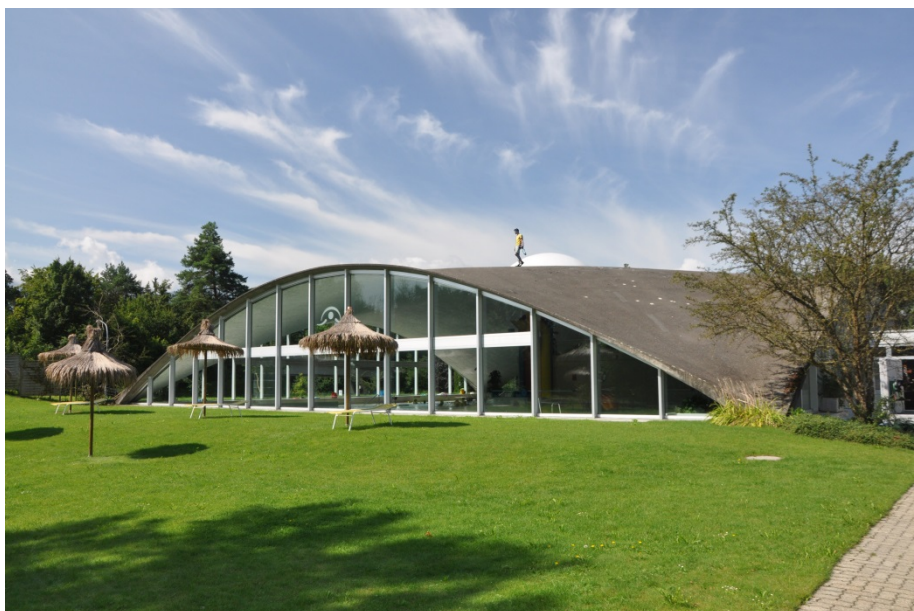
Figure 1: Swimming pool in Heimberg designed and engineered by Heinz Isler
