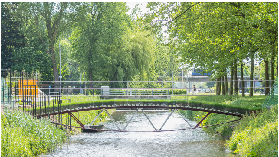
Figure 2: The Glass Truss Bridge. Note that the most left and most right diagonals are of steel. photo by Frank 'Graphdude' Auperle.
