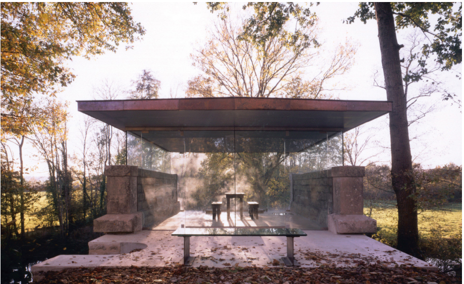
Figure 6. The temple de l' amour II in Burgundy (France) uses glass plates of minimal thickness to carry the compressive loads of the roof creating a full panorama (Kraaijvanger 2018).
