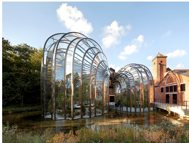
Figure 15a. Bombay Sapphire Distillery glasshouses extension in Whitchurch (United Kingdom) (Arkitecture 2015)
