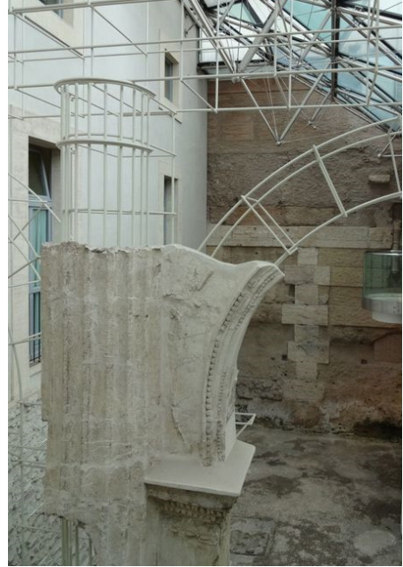
Figure 3b. Crypta Balbi's structural elements are restored with metal mesh (Rome, Italy) (Marigliani 2014).
