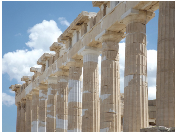
Figure 17c. Parthenon in Athens (Greece), built in the 5th century BC, is restored with the traditional technique of anastylosis in order to preserve the exact original shape and material (Barou 2016).
