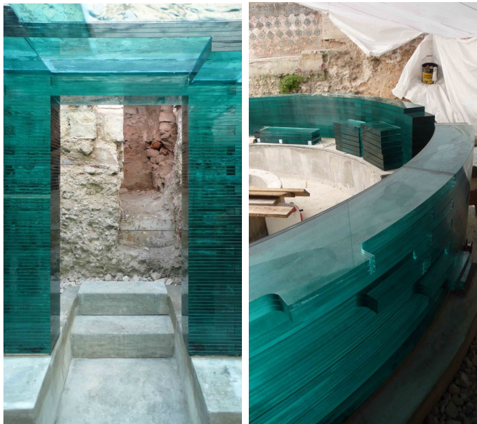
Figure 19b. The adaptive reuse of the Magdalena's fountain in Jaén (Spain) employing horizontally stacked float glass panels (Cuac Arquitectura 2018)
