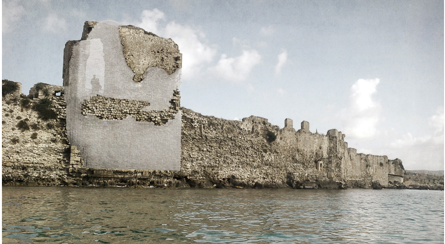
Figure 14. Restoration of the Bembo's Bastion by a glass masonry that consists of interlocking cast glass units. The glass structure fills the missing parts that have collapsed and completes the original shape of the tower (Barou 2016).
