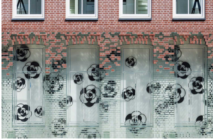
Figure 16. Detail of the Crystal houses façade in Amsterdam (The Netherlands) showing the transition of the glass-to-brick masonry with respect to the original construction technique ( https://www.archdaily.com/tag/prix-versailles )
