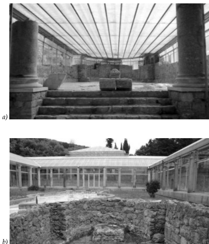
Figure 4. Restoration of Villa Romana del Casale in Piazza Armerina (Sicily) with a suspended transparent canopy made of glass and Plexiglas by F. Minissi (Vivio 2014)
