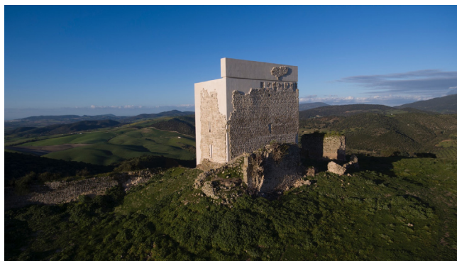
Figure 1a. The restoration of Martera Castle in Cádiz (Spain) has raised a big debate regarding the consolidation strategy, questioning whether the new limestone structure appears imposing on the remaining historic materials (Architizer 2015)
