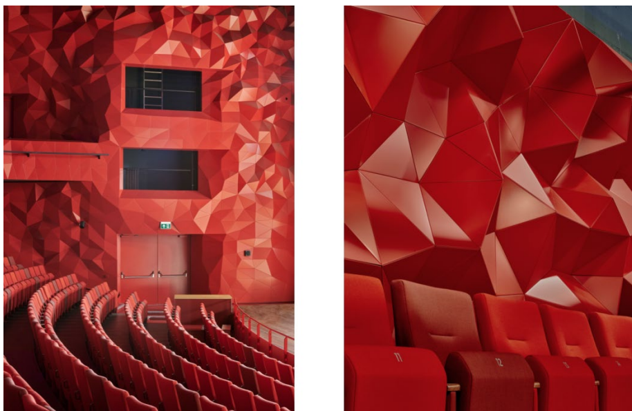
Figure 2. Flat areas of triangles and areas of triangles that form a folded surface, main concert hall Theatre Zuidplein, ©Studio RAP
