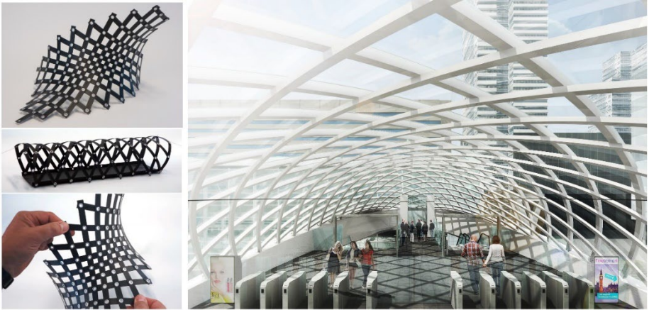
Figure 4. Physical prototyping of roof grid shell structure; Light Rail Station, The Hague(NL)
